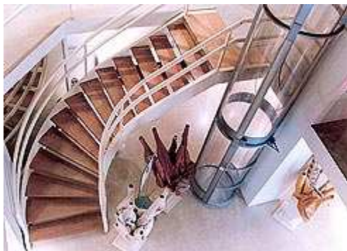
This pneumatic vacuum elevator uses suction to lift passengers.
